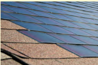
Amorphous thin film solar cells
