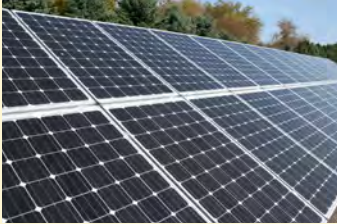
Monocrystalline solar cells
